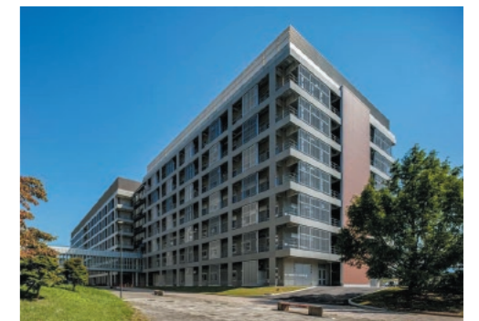
Biomass Green Innovation Center (established in 2022)
